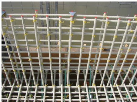
Headed V-ROD® in deck and barriers
