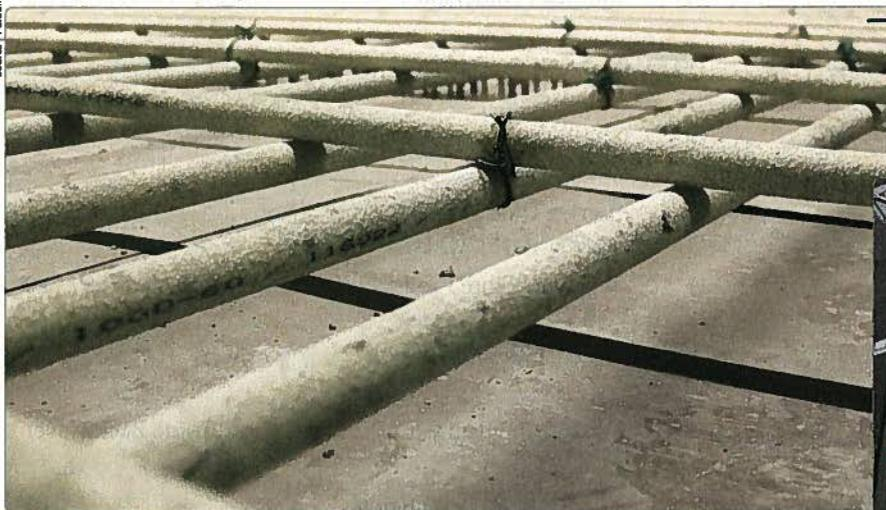
Composite rebar, like the V-ROD product from Pultall shown here, replaced steel rebar in reinforced concrete poured for the first-floor slab during rehabilitation of La Chancelière parking garage (inset) in Quebec City. ■
