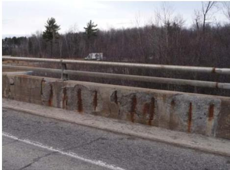
Fig.1 Corrosion-induced degradation of steel-reinforced bridge barrier wall
